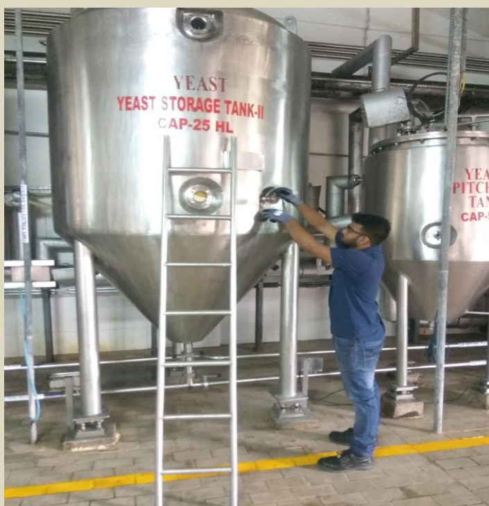
Figure 12: Yeast Storage Tank
