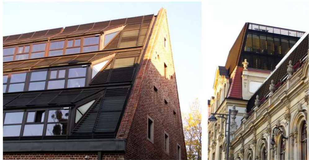
Figure 4. Contrast to underline the border between the old and the new (to emphasize historic character of the building), (left) The Granary Hotel, Wrocław, (right) The Hotel Monopol, Wrocław.
