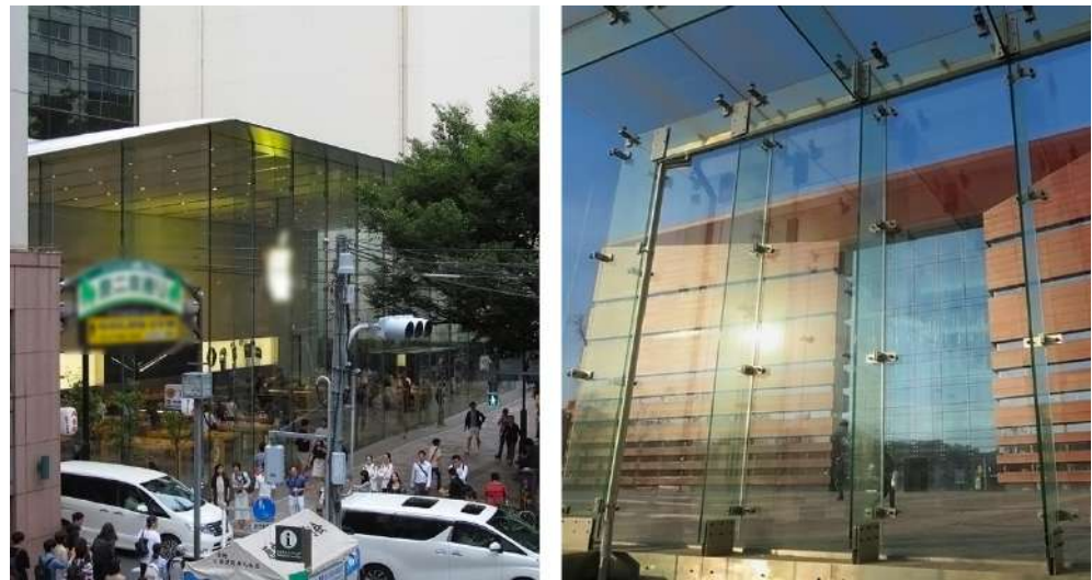
Figure 2. Transparent facade solutions—full interior-external visibility, (left) The Apple store in Tokyo, Omotesando, (right) parking exits pavilion at the Plac Wolności, Wrocław (in the background The National Music Forum).
