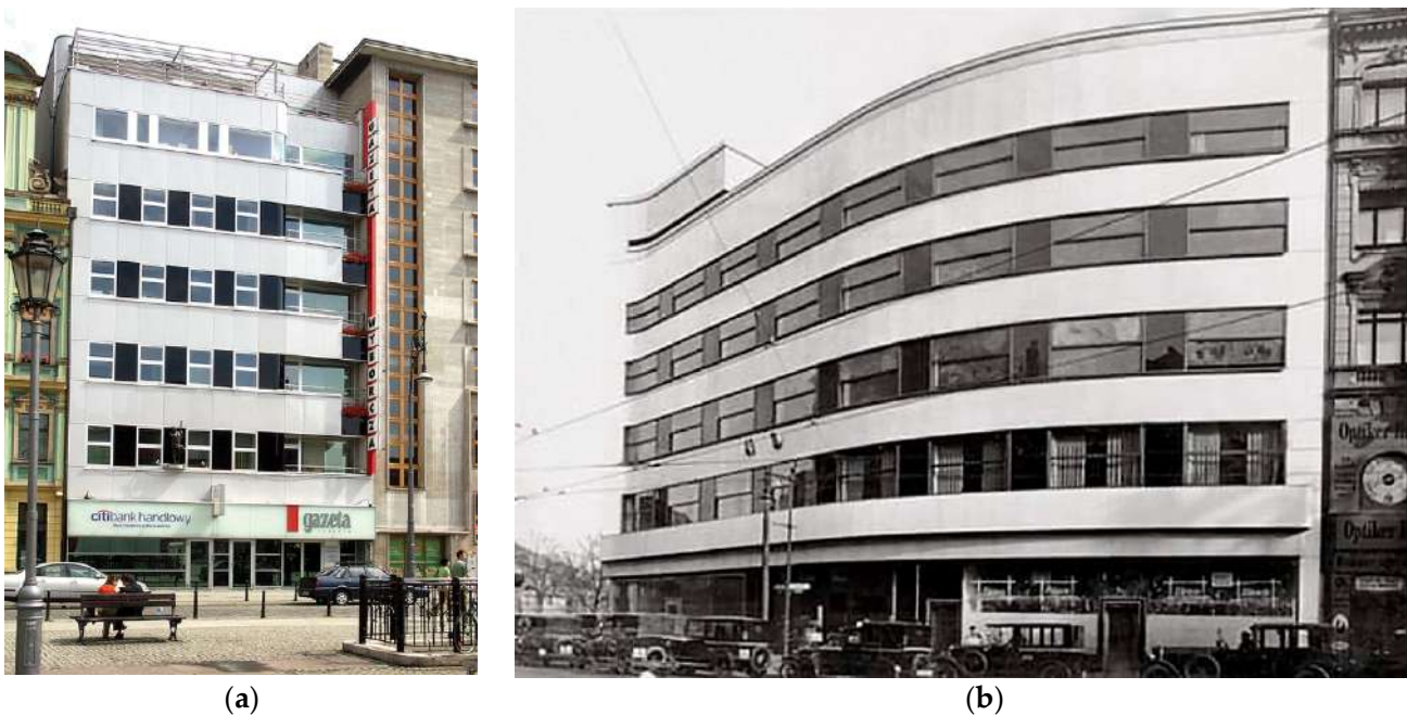
Figure 3. (a) The Geschäftshaus Mohrenapotheke at 2/3 Solny Square Wrocław, Adolf Rading, performed in 2004; Photo by, Andrzej Krupa (b) The Teleschow-Haus at Potsdamer Platz Berlin, 1927, arch. Brothers Luckhardt and Alfons Anker. Both buildings had their facades built using Opakglas. Archival photo Max Krajewski.
