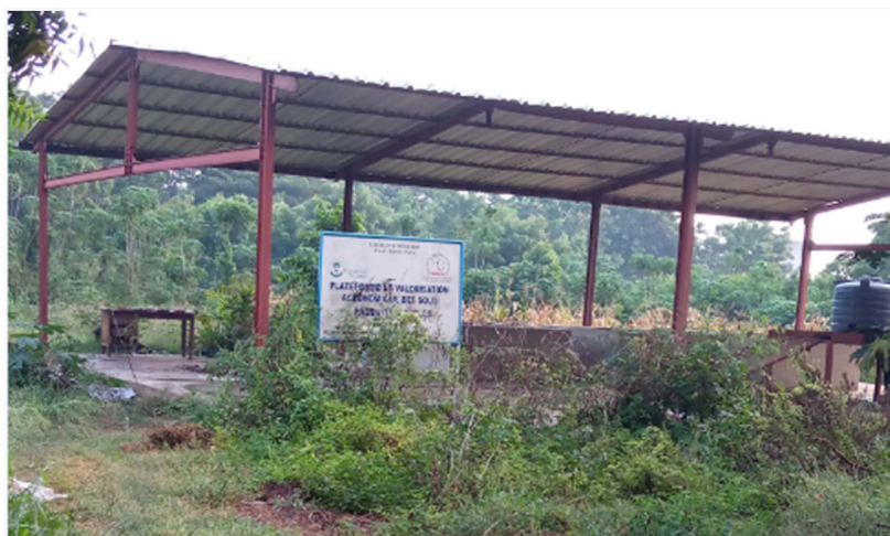
Figure 1. Photo of the worksite.
