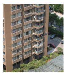
**Figure 5.** High-rise apartments, Ningbo block H: inappropriate climatic design with only a few of the apartments facing south and less opportunities for cross-ventilation, double-sided ventilation, and natural lighting (source: the authors).
