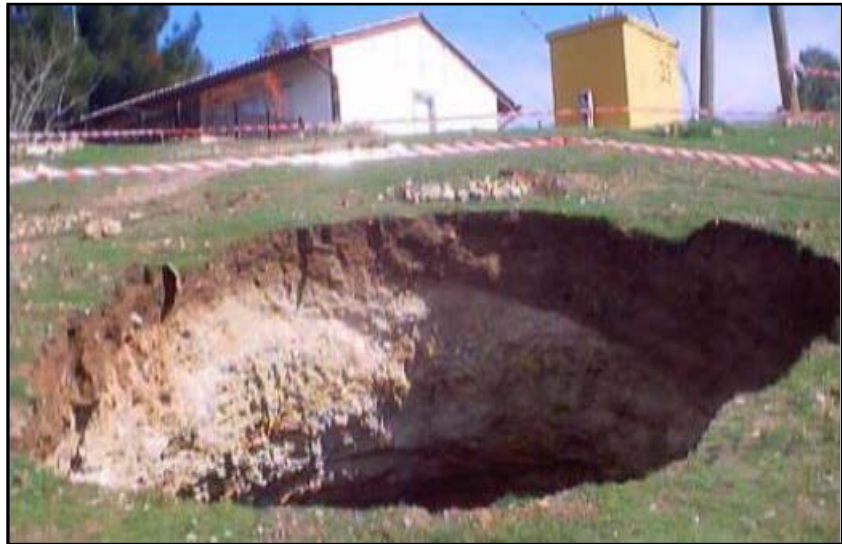
Figure 4. A sinkhole which was developed downstream after filling the reservoir (15 February 2015)
