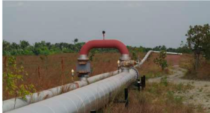
Figure 1. Loop in pipelines of heavy crude oil.
