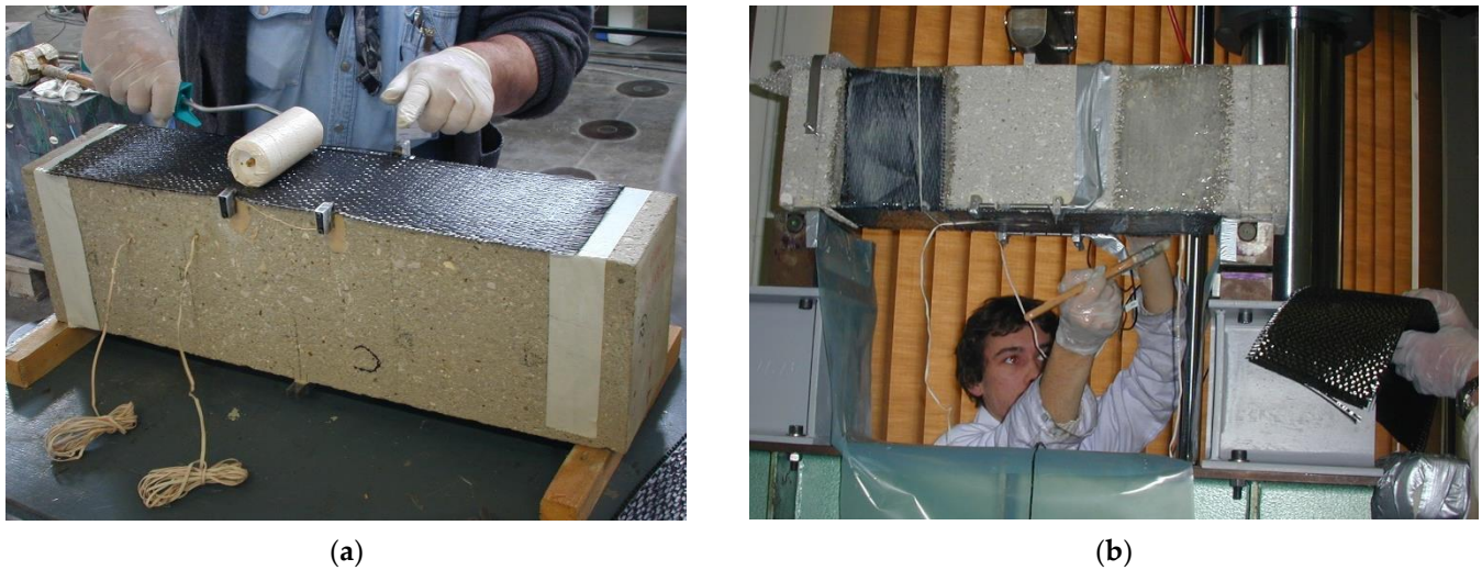
Figure 6. Strengthening of specimens: (a) beam ES1 positioned upside down; (b) CFRP strips bonded as in the field (technicians working under the beam ES2).
